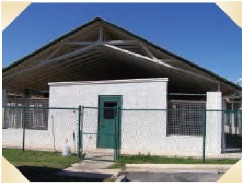
The roof-over-roof design helps keep fresh air flowing through the boarding areas.
